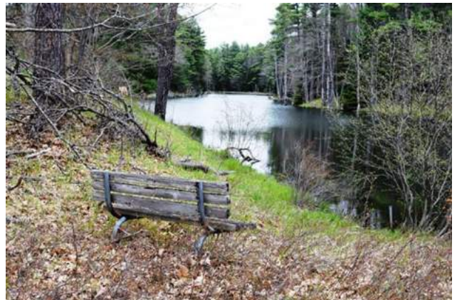
Picnic Pond Stormwater System is located at the former Brunswick Naval Air Station.
