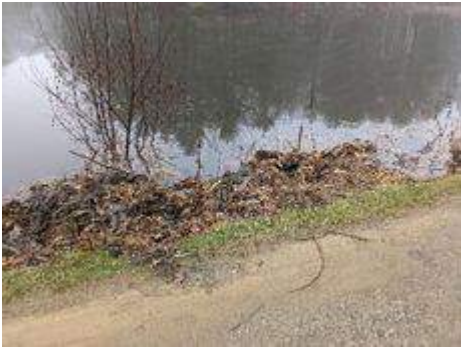
cul25 Inlet Pipe
