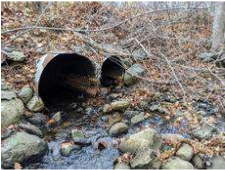
cul10 Outlet Pipe
