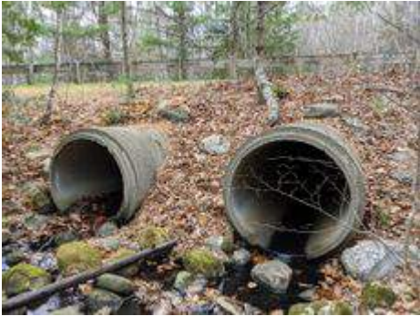
cul03 Outlet Pipe
