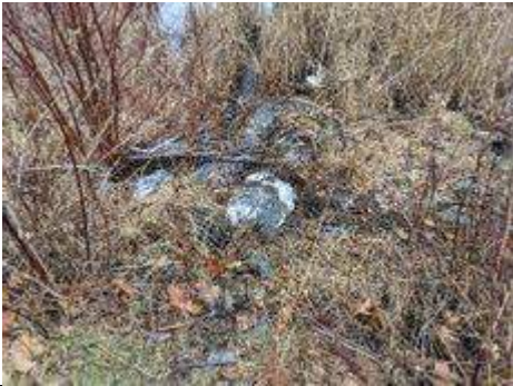
cul25 Outlet Pipe
