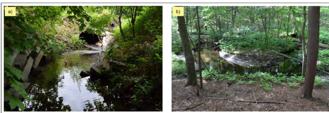
Figure 11. Reach 9 is a) narrowly confined and undermining granite blocks on the bank at the outlet of the Maine St. culvert but b) has a sinuous planform with abundant wood in the channel downstream.
