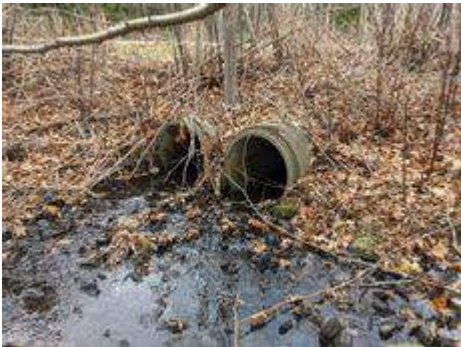
cul05 Outlet Pipe
